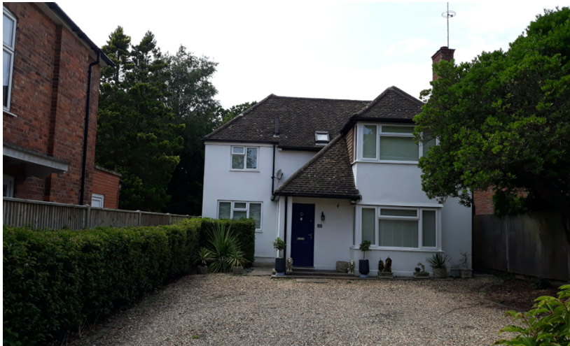
Photo of the rear elevation of the application site
